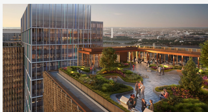
Rooftop Terrace - Eight of Met Park's 19 landscaped terraces will be actively programmed, with amenities ranging from outdoor meeting spaces and dog runs to an urban farm.
